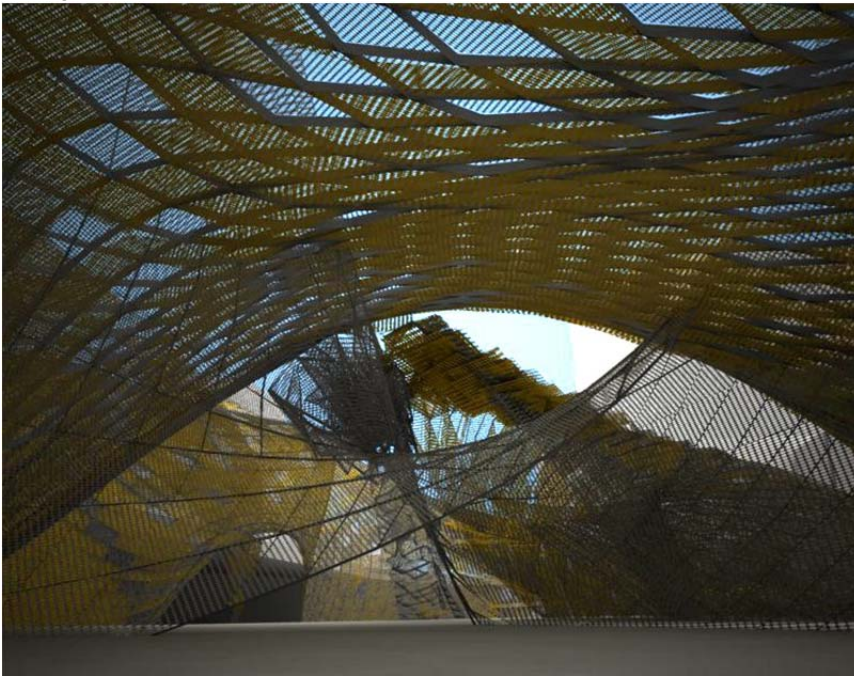
Figure 14: The grating ensures a degree of lightness while providing elemental filtration for a large structure that could otherwise be quite oppressive
